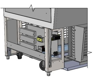
View of Ballasts (After Removal of Electrical Box Cover)
